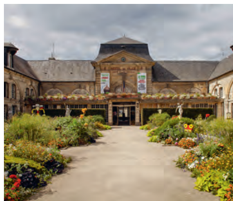
Town Hall, Stains
